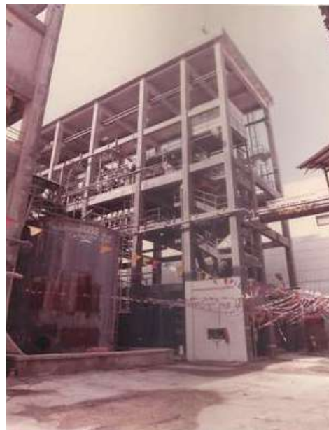
MAIN BELT FILTER BUILDING
